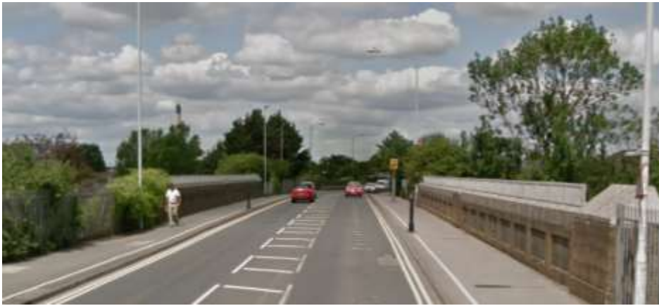
Farnham Road Overbridge Approx. 35m in length, Bollards 7m <> and speed camera.
